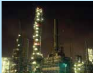
Sohar Aromatics Plant-civil works for Oman's first Aromatics plant
