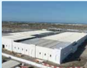
A'Seeb wastewater Treatment Project for Haya Water
