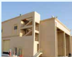
Civil works for Dubailand 2- Sub Station project in Abu Dhabi
