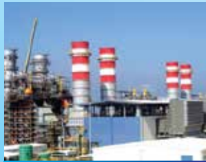
Sohar Aluminum Smelter-1000 MW Captive Power Plant in Oman
