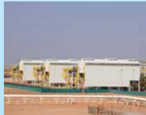
Saih Nihayda Depletion Compression Project for PDO and GS E&C
