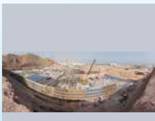
Emergency Water Storage Reservoirs project for PAEW
